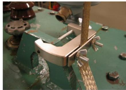
Place the braid between the G-clamp and the braid plate. Tighten the braid to create a straight line from the C-clamp to the G-clamp. Tighten the wing nuts.
