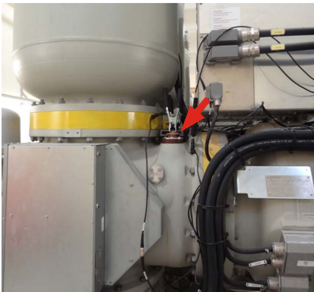
One of the ferrites (C plus I) on the copper bus.
