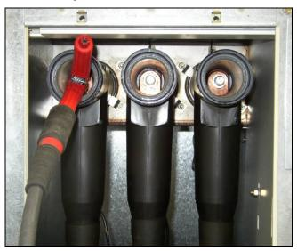
For this connection situation, the optionally available connection set (see section 2.3.1) provides a suitable adapter used to directly plug the connection cable on the MC connector:
