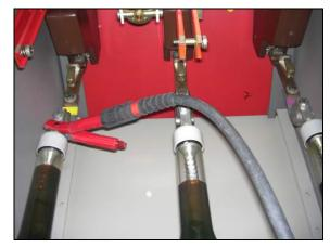
In particularly tight situations (such as in the following shown substation), one can undertake suitable protective measures to avoid a flashover. In this case, a semiconducting rubber mat was laid between the connection cable and the metal edge. Another point to be aware of is the connection to the phase. Special care should be taken here to ensure a PD-free connection.
