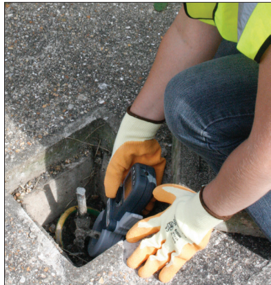
The Megger DET14C shown measuring a ground spike in a typical ground well.
