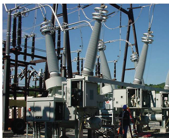
Dead tank circuit breaker
