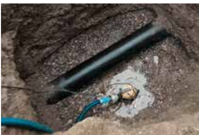
Cost-effective installation without chamber construction
